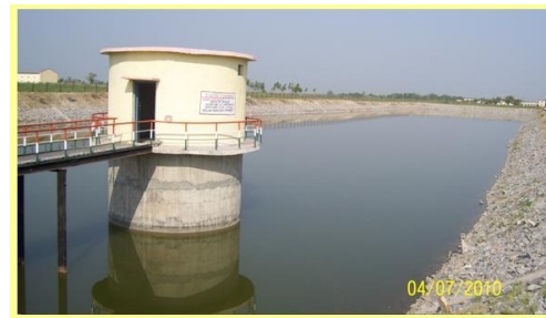
Jack well-cum-pumphouse in reservoir in Karnataka
